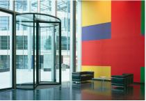
The east entrance at Tower Place in london was designed by architects Foster and Partners. This installtion is a fully automatic **record K41** four wing revolving door and has an all-glass drum with visible parts anodised. The operating drive for this revolving door is concealed beneath the floor in a casing which protects it from water and dirt.
