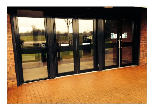
This is the entrance to the Stepps Pavillion at the University of Strathclyde in Glasgow. The doors on the right hand side are a pair of **record low energy swing doors** (DFA 127 LOW ENERGY) providing slower opening for disabled access. The middle doors are manual swing doors.
