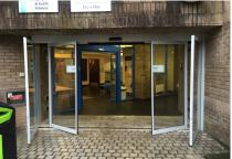
Geographical and Earth Sciences Department in Glasgow University. This is the record TOS - Total Breakout system which is a sliding door with break out capacity suitable where emergency passage may be required.
